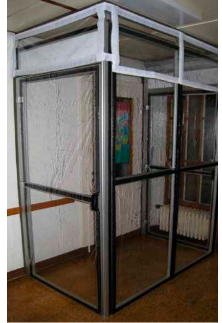
Double door system for dust protection
